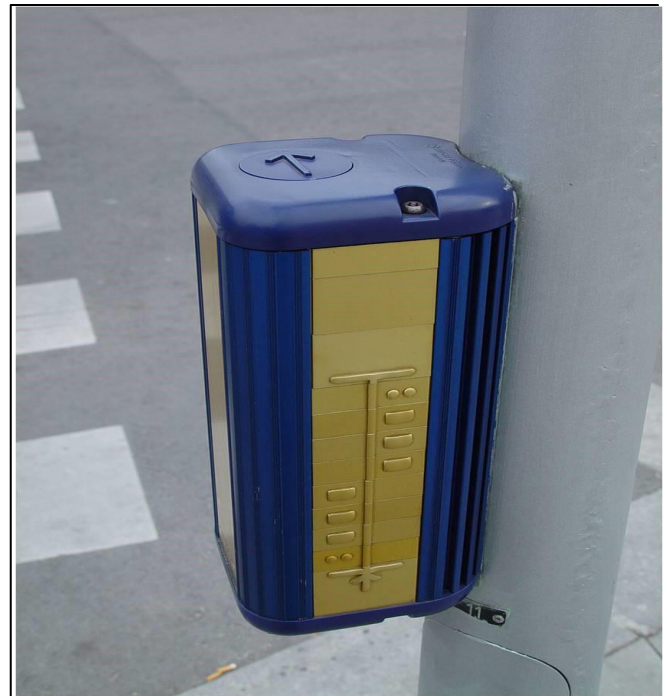
Photo of a pedestrian crossing with a push button that incorporates a tactile arrow to indicate the direction of crossing and a tactile map showing the lane configuration along the crossing route.
